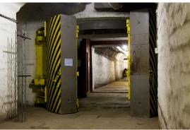
**manufactures and renovates** anti-pressure and gas-tight doors, hatches and closures. These are designed with a back pressure resistance of 200 KPa and higher. We also produce doors and hatches in ballistic resistance FB4/BR4, FB6/BR6, TBO3, TBO6 according to ČSN 395360.
